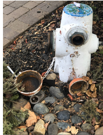
Fire department employees encountered a yellowjacket nest at the base of this fire hydrant.
