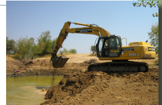
Construction of a Sacramento Perch recovery pond
