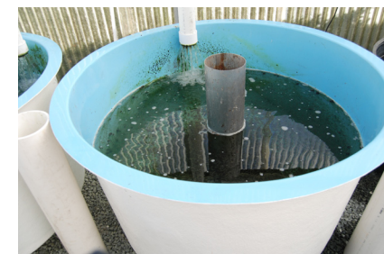
Cool water holding tank
