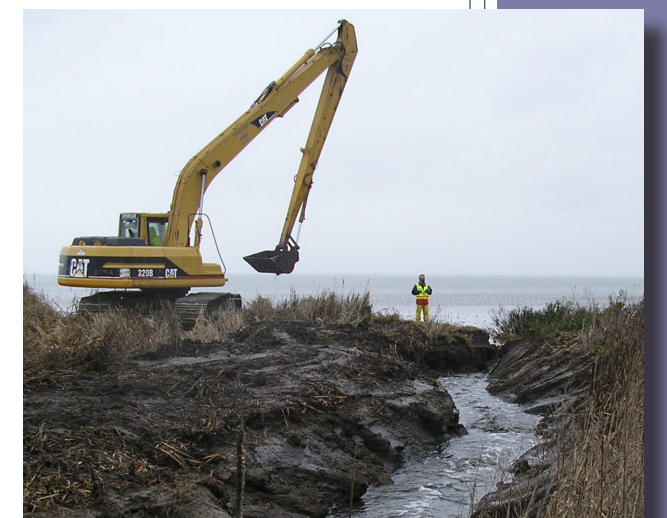
Long-reach excavator clearing tide marsh channels
