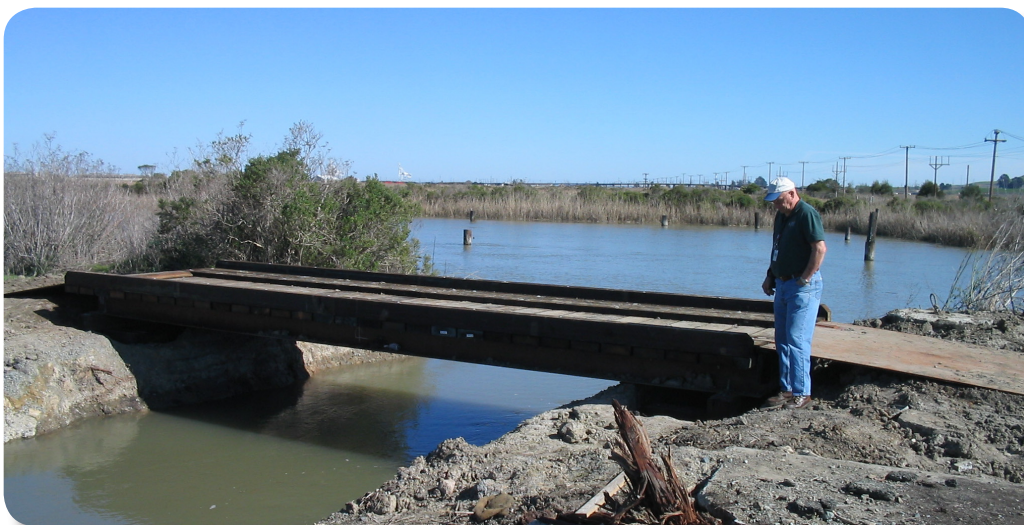
Fig. 2. Bridge over new tidal channel, Concord Naval Weapons Station
