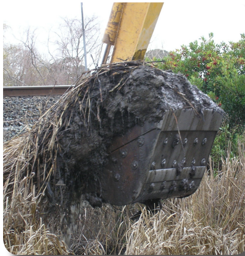
Fig. 1. An excavator clearing a drainage channel in Tara Hills
