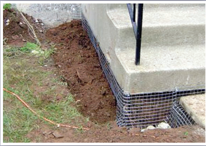
L-Shaped screen application around foundation**
