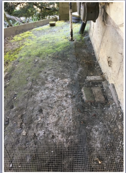
Above ground screening using concrete screw anchors and galvanized garden stakes
